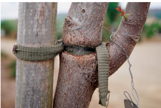
Figure 13: An example of tree tie damage in which the support tie has constrained growth of the trunk.
